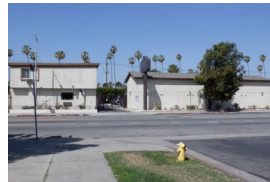
Western Avenue Apartments
