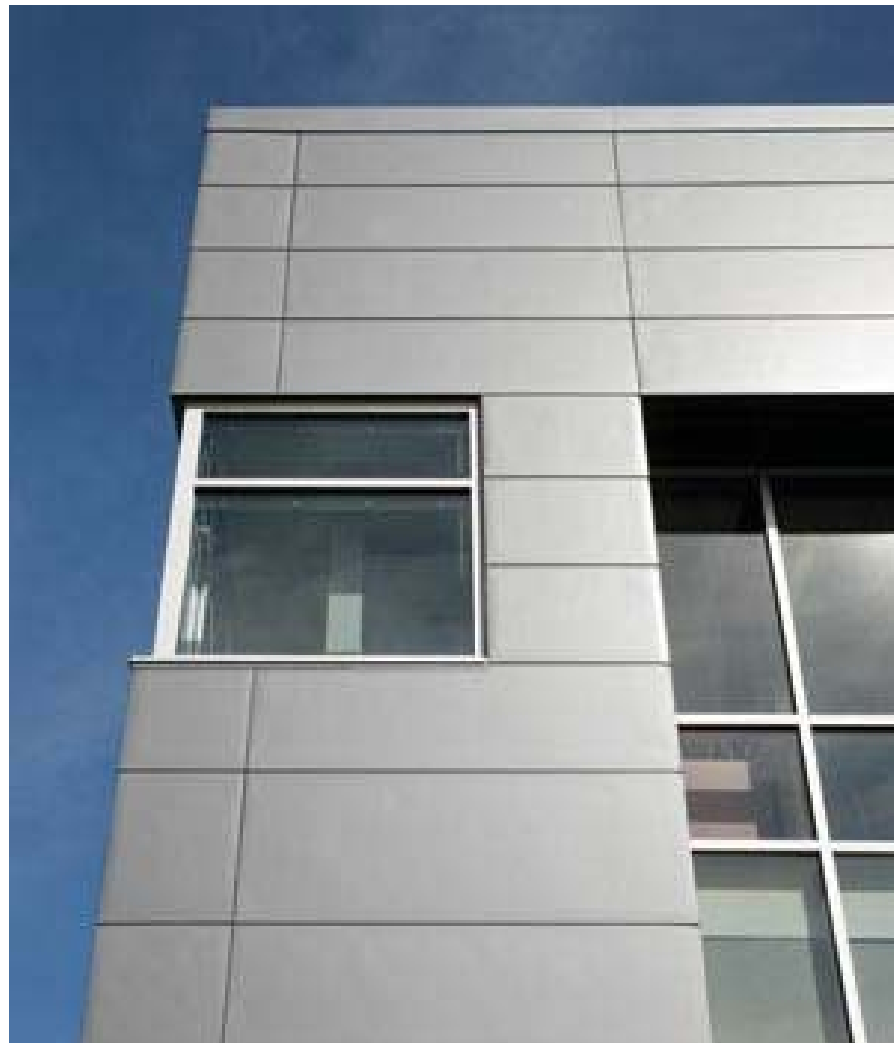
ALUCOBOND VERTICAL COMPOSITE METAL PANEL
